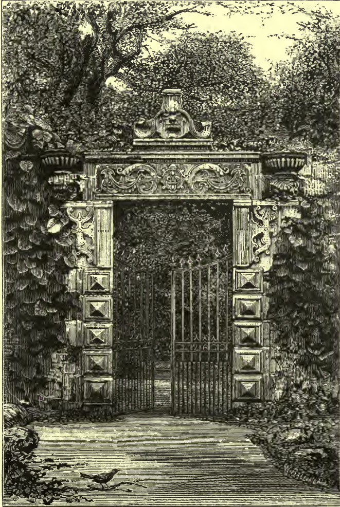
GARDEN GATE BUILT OF STONES FROM THE OLD PARLIAMENT HOUSE (except the Mask on the top).
